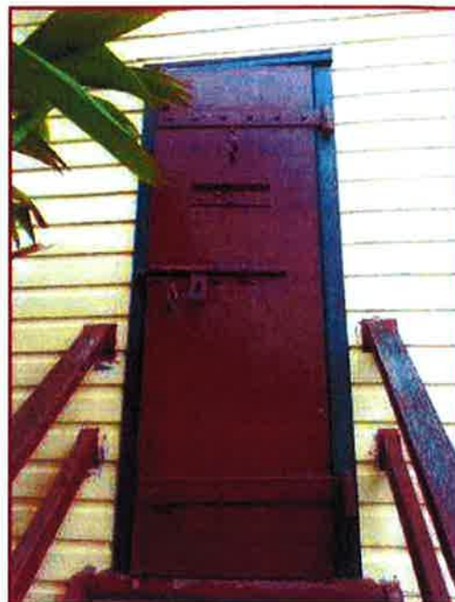
Figure 3.12: Door to the lock up (Clarence Valley Council).
