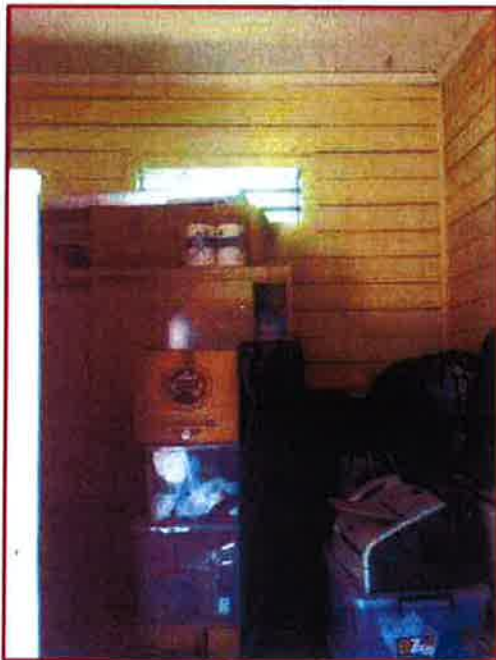
Figure 3.11: Interior of the lockup room with small, horizontal barred window (Ainsworth Heritage).
